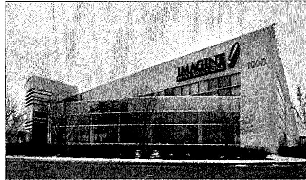
Imagine! Print Solutions of Shakopee plans to break ground this year on a 300,000-square-foot addition to its roughly 500,000-square-foot headquarters — one of three major industrial-related construction projects planned in the southwest Twin Cities suburb. (Staff photo: Bill Klotz)
